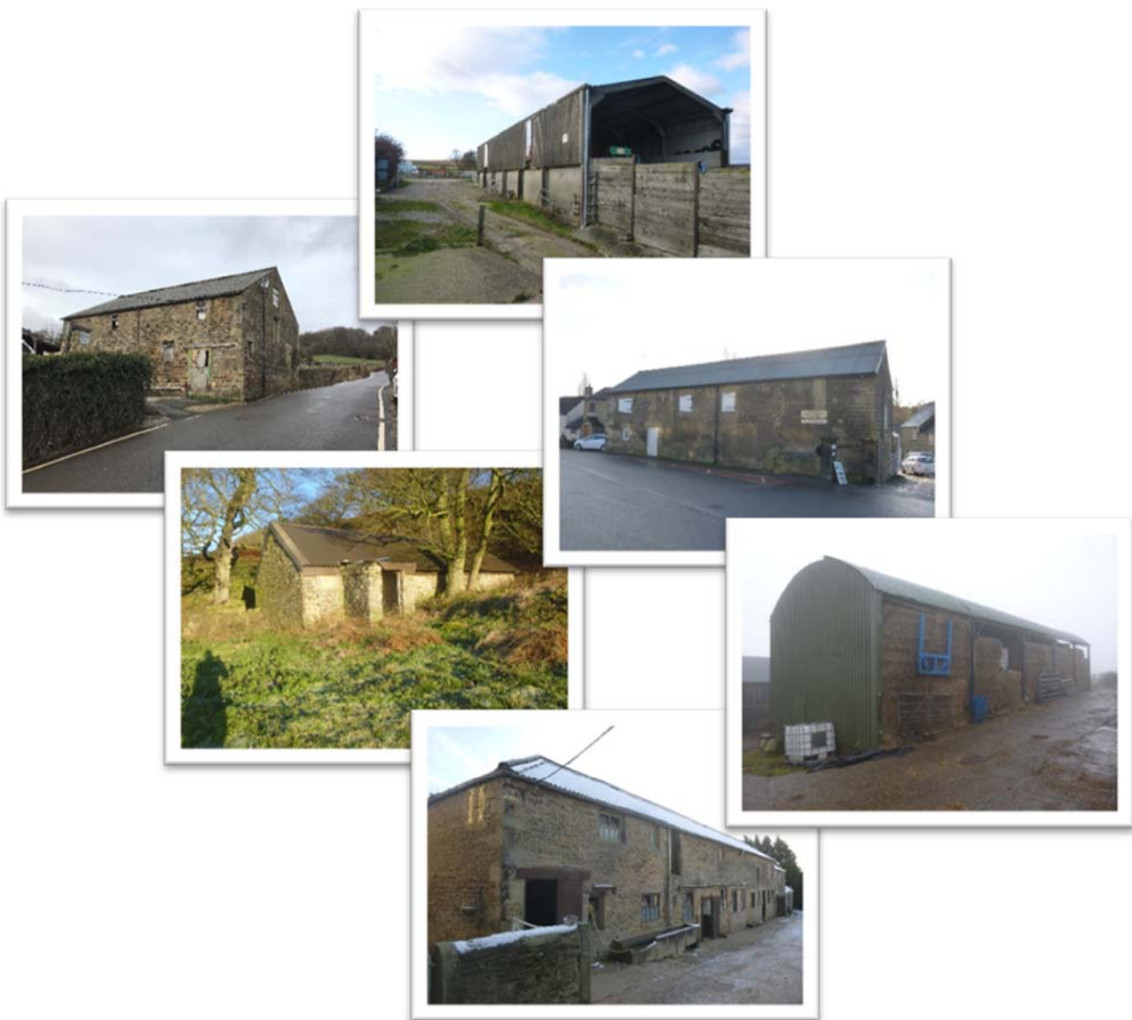
Figure 5: Examples of buildings on the Rural Estate
